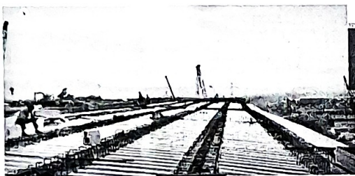
DECK SHEET LAYING FOR DECK SLAB
