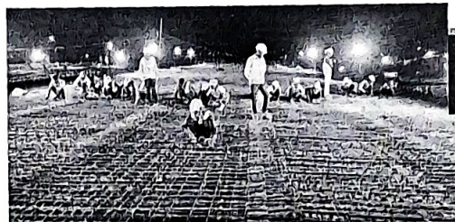
REINFORCEMENT TYING FOR DECK SLAB
